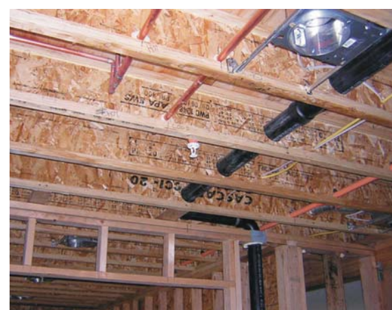
Inspecting new residential construction
